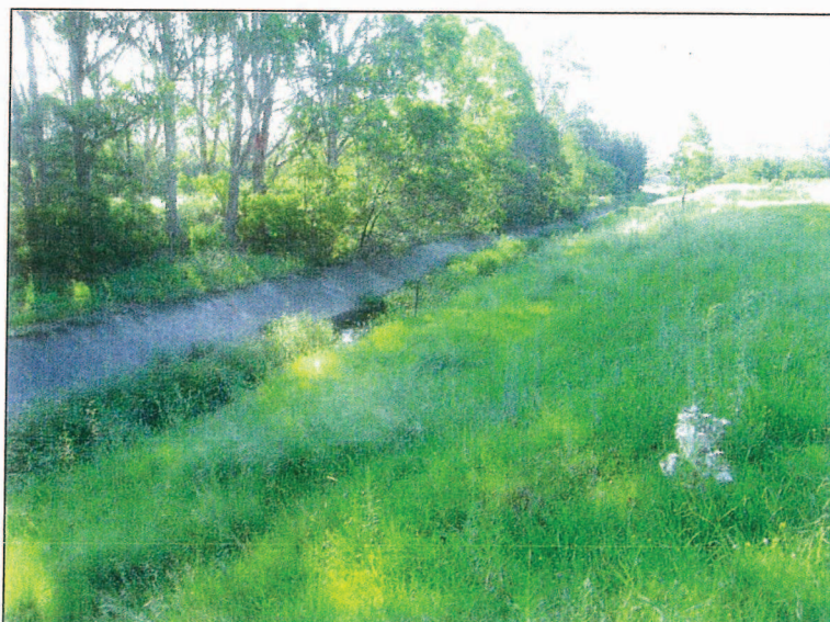
Photograph 12: Looking across from the northern bank of the canal to the southern bank southern bank planted with native vegetation whilst the northern bank is grassed)
